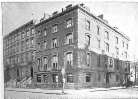
CALUMET CLUB, FIFTH AVENUE AND EAST 20TH STREET.
